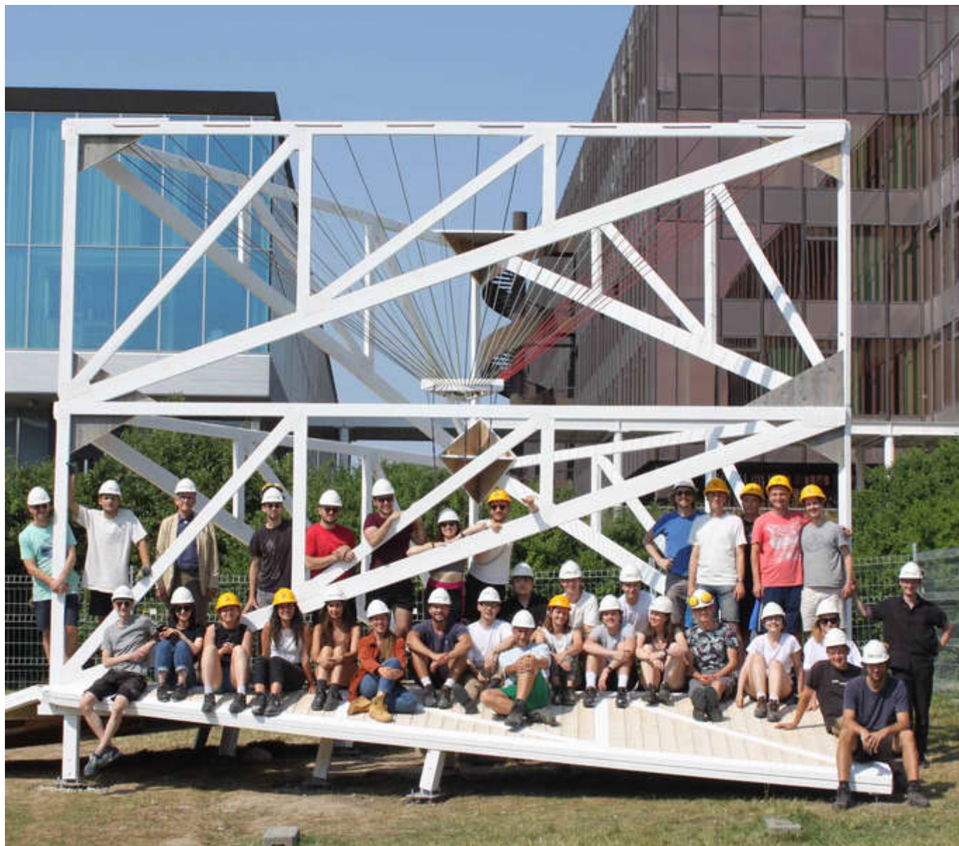
Construction of a structure designed by students with reused materials from the Huber Pavilions on the ETH campus.
