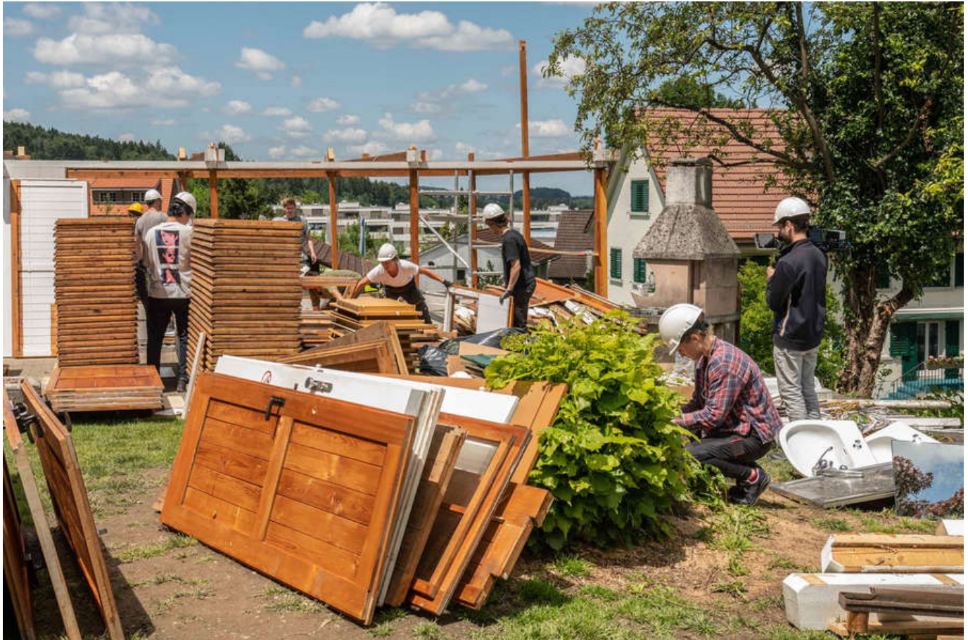
Disassembly of the Music Pavilion near Zurich by the students of the Digital Transformation for Circular Construction course by Prof. De Wolf.
