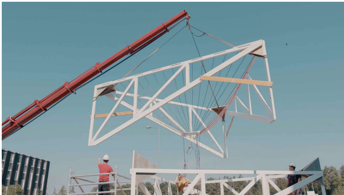
Assembly of a structure by the students of the Digital Transformation for Circular Construction course by Prof. De Wolf with reused trusses from the Huber Pavilions.
